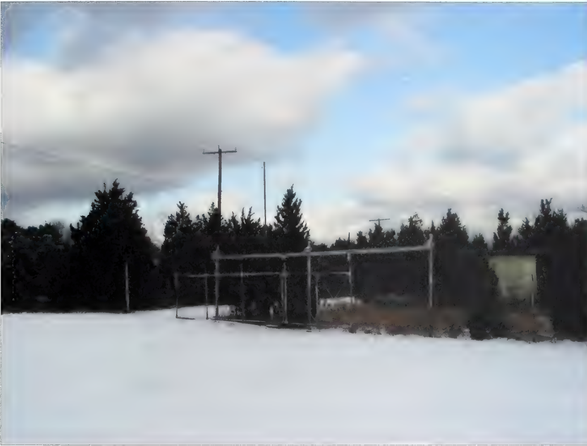
Figure 4.26. View looking northeast at access gate to Missile Magazines and Missile Maintenance Area, NIKE launch site. Following the site's closure woody species, especially eastern red cedars, have emerged and are growing in close proximity to the buildings. The Paint and Oil Storage shed (447) can be seen on the right foreground surrounded by eastern red cedars (Olmsted Center, January 2009).
